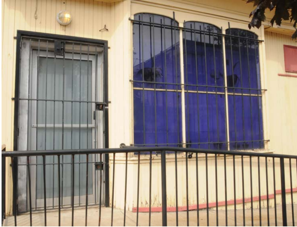
Locked emergency access to Gosnell's clinic
