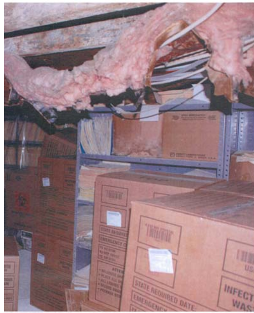
Boxes of bio-hazardous waste in basement
